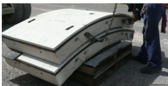
Bottom: Segment placed into the lifting frame (underpin installations)
