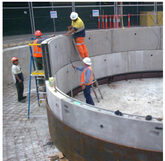
Step 6 – Constructing first ring on top of bottom/choker ring segment
