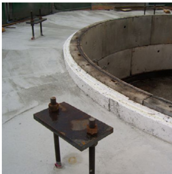
Step 11 – Jacking gallow anchors in place
