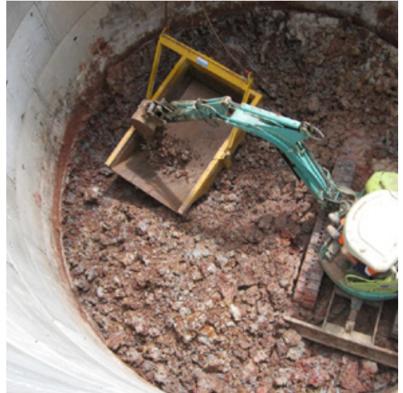
Step 13 – Excavation inside the shaft
