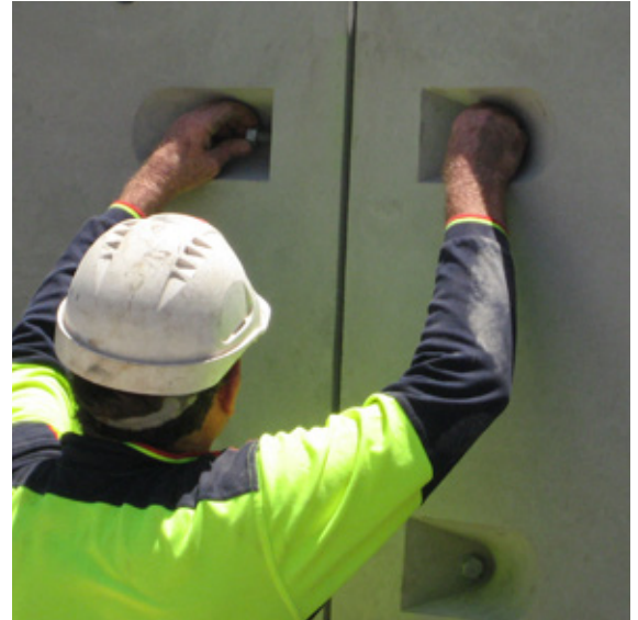
Step 10 – Fixing the curved bolts
