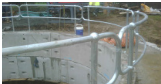
Step 4 – Guardrails in place
