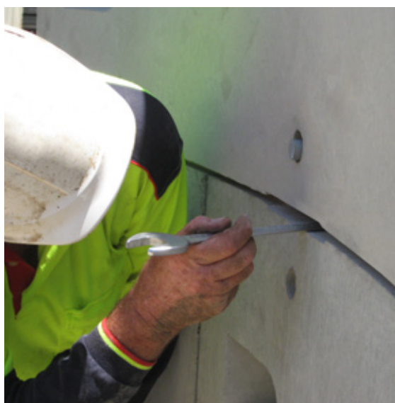
Step 9 – Tightening the joints
