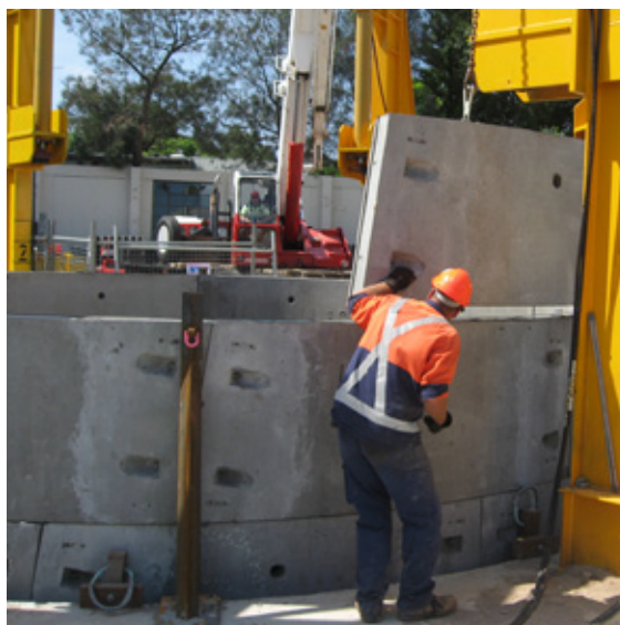
Step 12 – Top ring acting as a safety barrier
