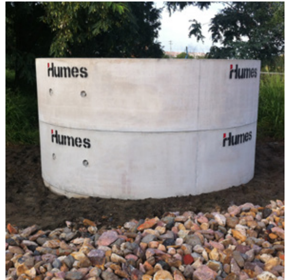
Complete one piece shaft installation
