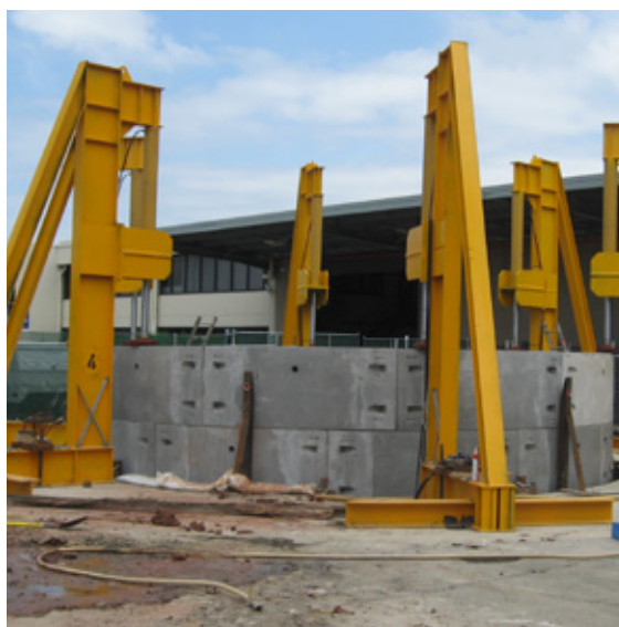
Step 11 – Jacking gallows in place
