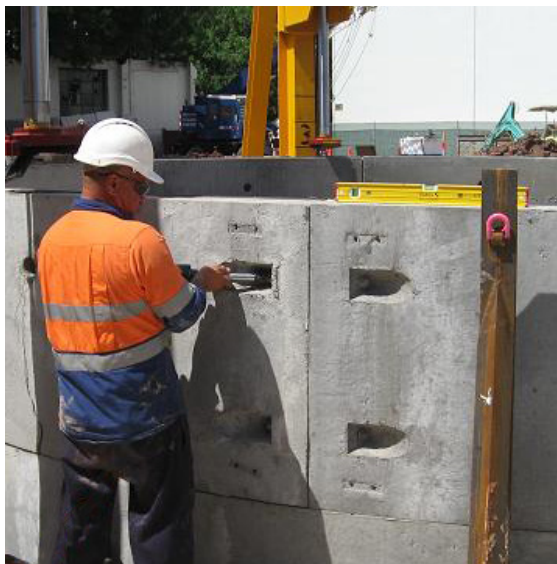
Step 7 – Making vertical joints using curved bolts
