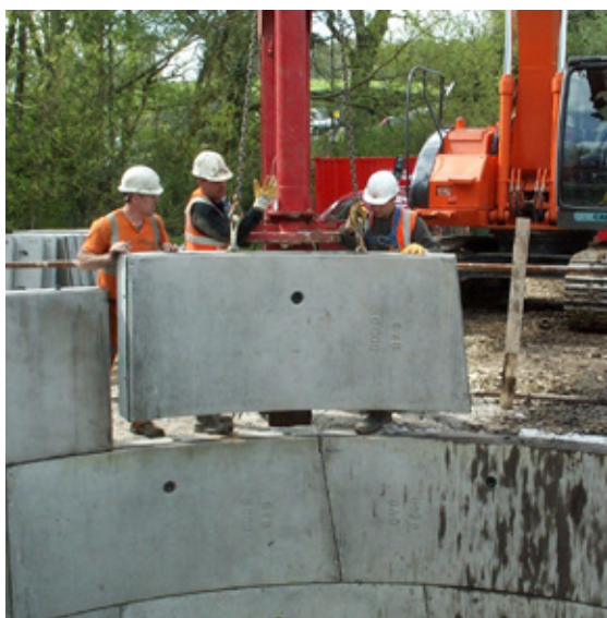
Step 8 – Installing the tapered segments
