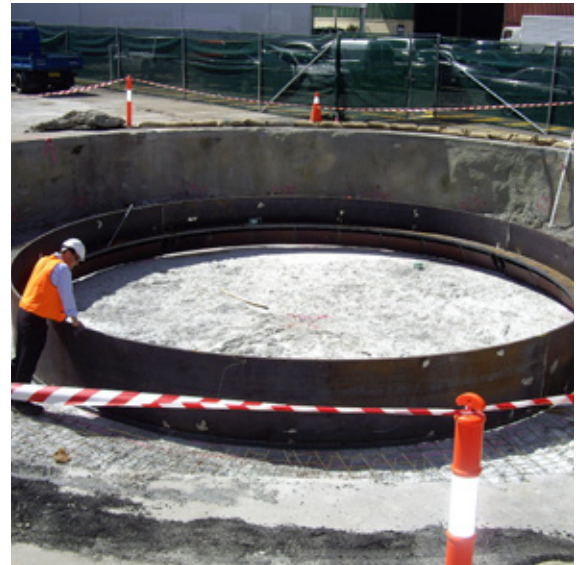
Step 2 – Completed steel cutting edge
