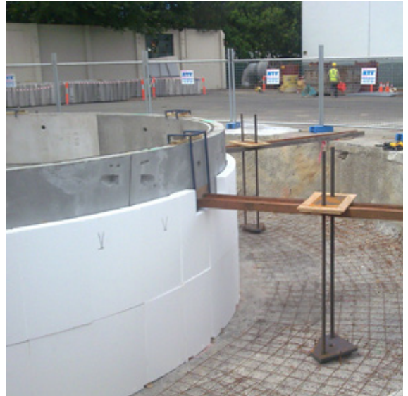
Step 9 – Surrounding ring with polystyrene to create an annulus
