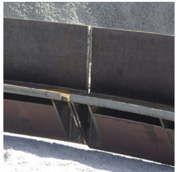
Step 2 – Detail of steel cutting edge
